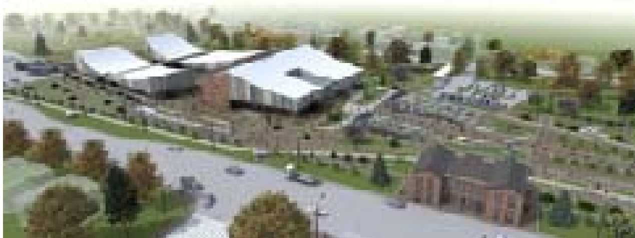
Ill. 8. Museum complex on Lychakivska str. – general view, edited by A. Pizhovska, 2013
