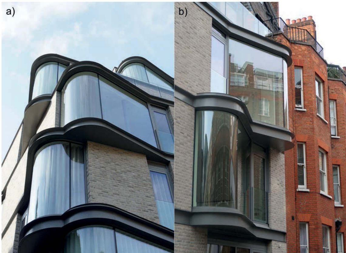
III. 9. Residential building on Castle Lane in London: a) bent glass in facade, b) bow windows. Photos by A. Józwick, 2019.
