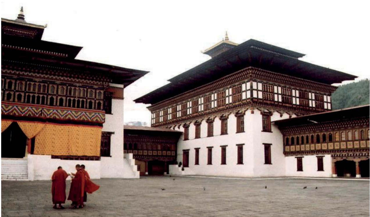
III. 3. The form of the roof communicates the important function of the building. Bhutan, stacked pent hip and hipped roof over a religious and administrative facility. Photo by K. Sobczyńska (Sobczyńska, 2012, p. 124).
