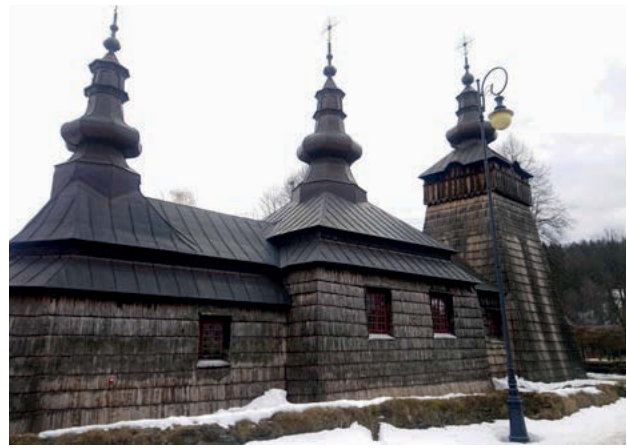
III. 2. Stacked roof over a religious building, Poland, Orthodox church in Szczawnik. Photo by K. Sobczyńska.
