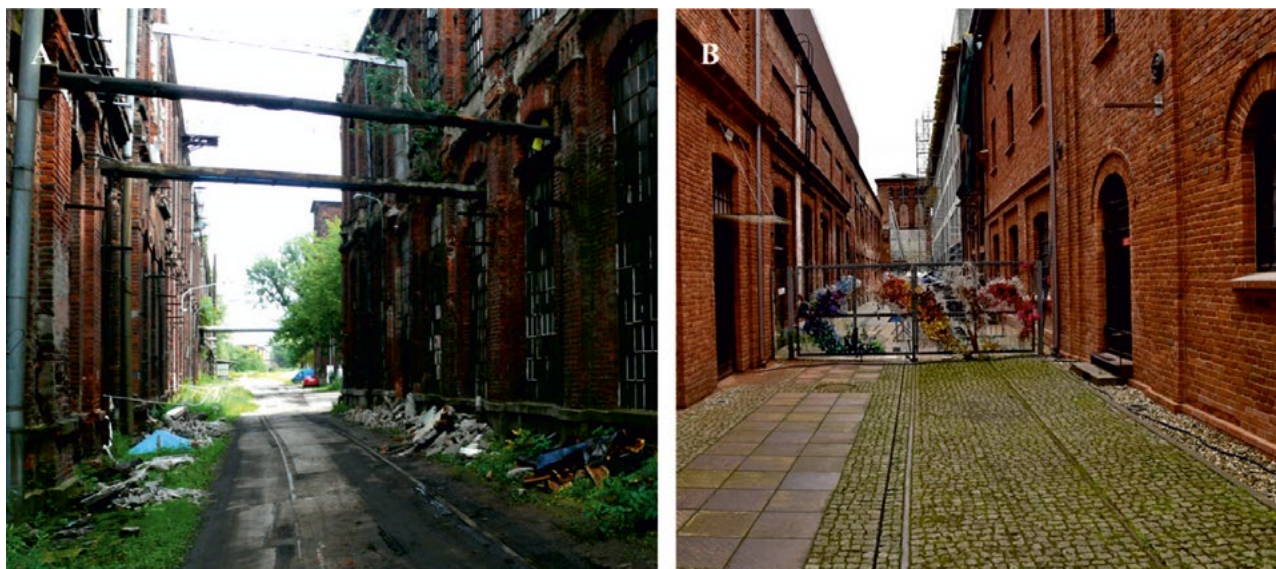
Ill. 10. The course of the Schiebler railroad. A) The defunct railroad at the Scheibler complex (2017). B) Use of the railroad in the pedestrian walkway space at Art-Inkubator (2023). Photos by A.A. Tomczak.
