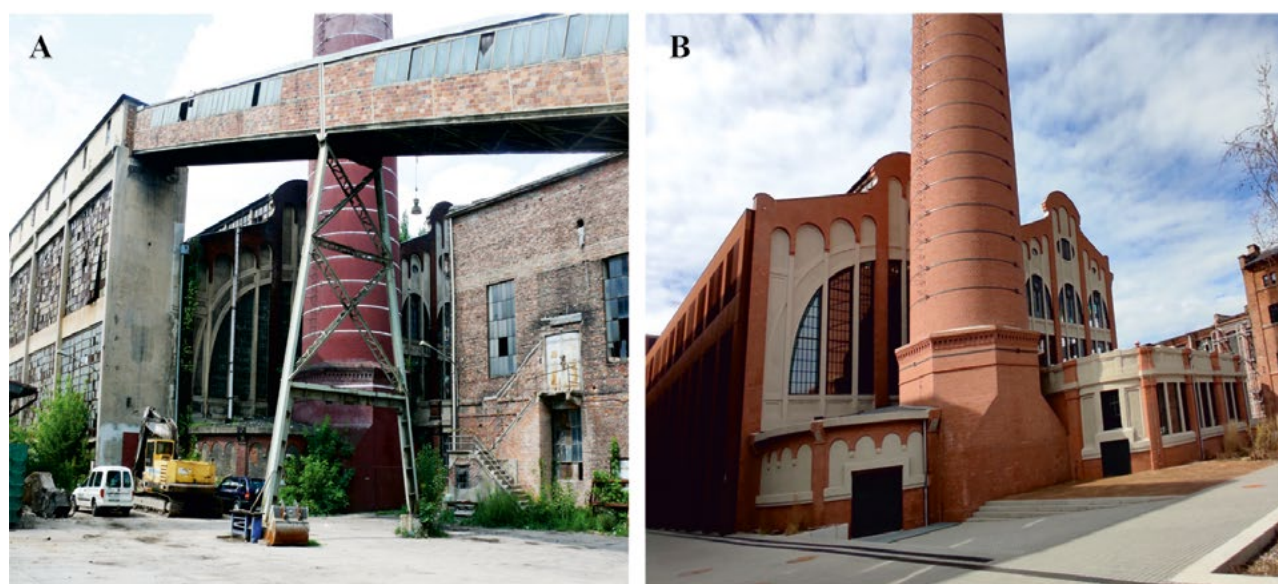
III. 8. Exposure of the front elevation of Scheibler's power plant. A) State of preservation (2017). B) The building after renovation with introduced recreational and cultural uses and developed a forecourt (2023). Photos by A.A. Tomczak.
