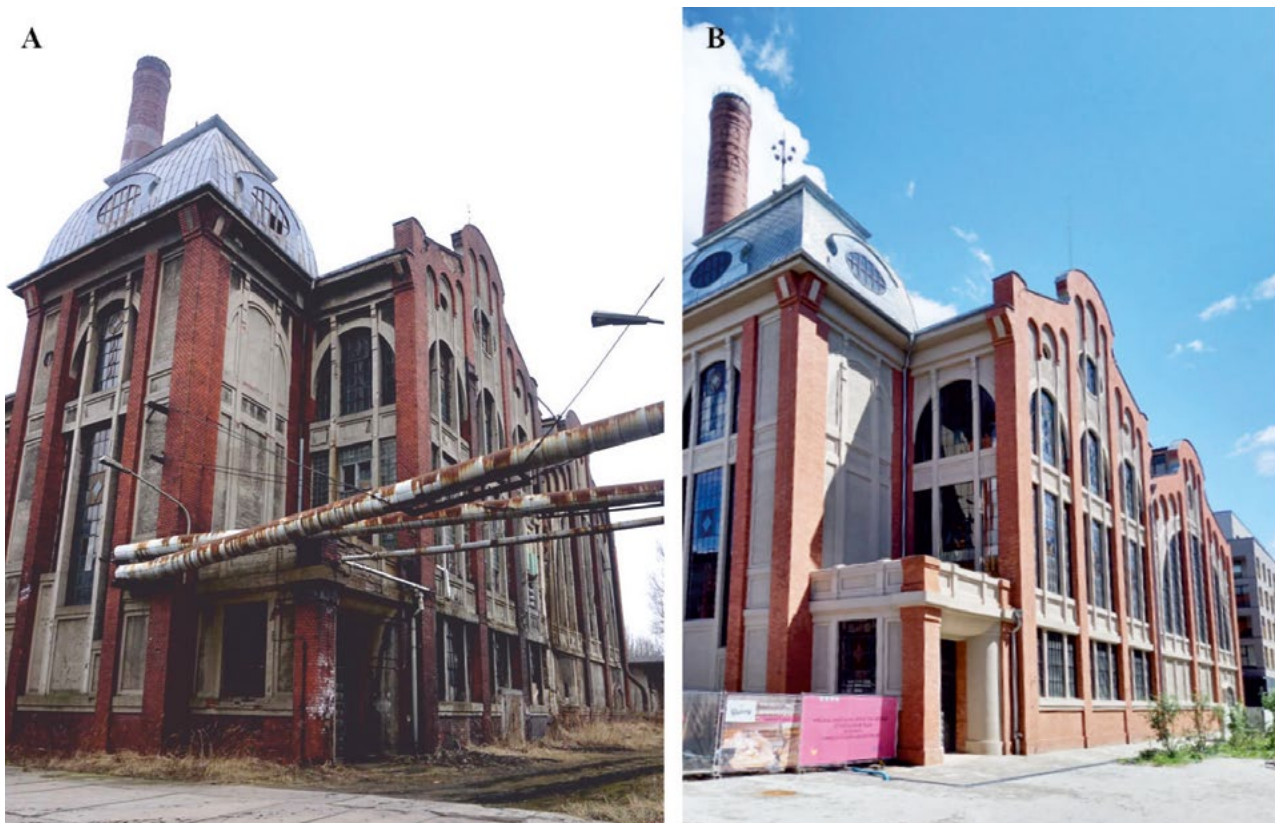
Ill. 9. Karol Scheibler's Art Nouveau power plant from 1910, built to a design by Alfred Firsch. The oldest building within the borders of the then Kingdom of Poland in reinforced concrete frame construction. A) State of preservation (2017). B) As seen after the revitalization (2023) Photos by A.A. Tomczak.
