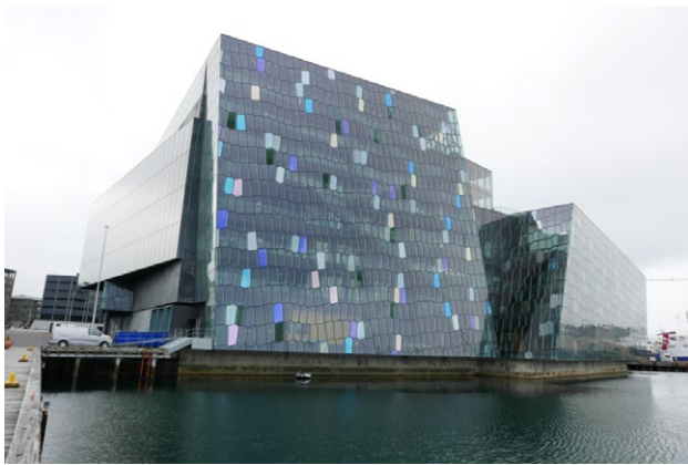
Ill. 3. Harpa, proj. Henning Larsen Architects, 2009. Photo by the Authors, 2021.
