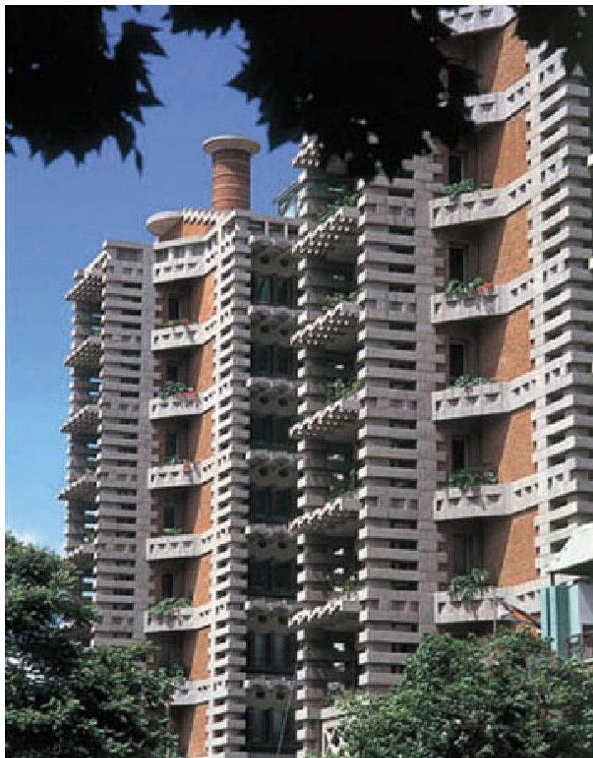
Ill. 3. Eastgate Building in Harare.
