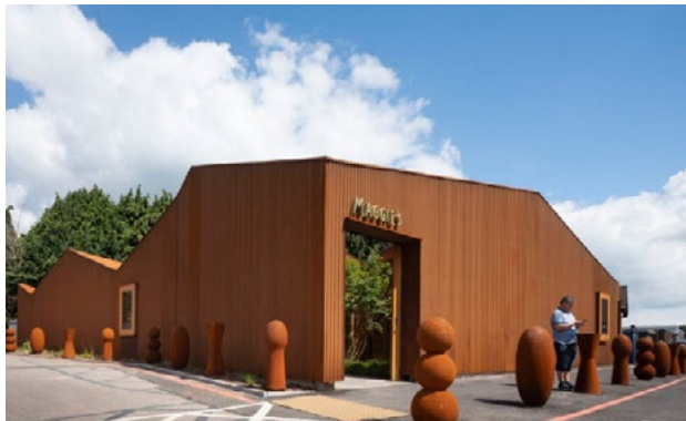
Ill. 8. Maggie's Centre Hospice in Cardiff (Dow Jones Architects, 2019).
