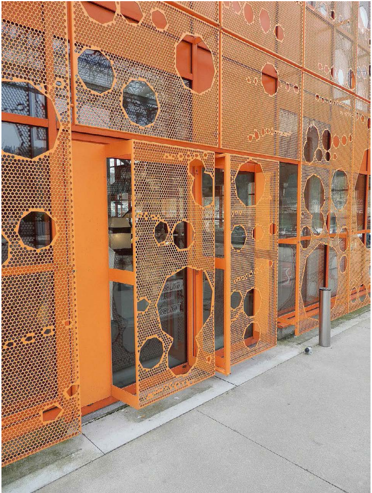
Ill. 3. The Cube Orange building — detail of the metal exterior shell. Photo by W. Kosiński, 2017.
